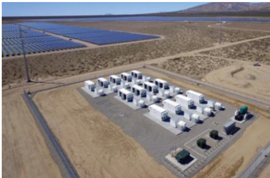
Figure 1: A 20MW/10MWh containerized BESS combined with 570MW of solar PV (source: ccj-online.com)
