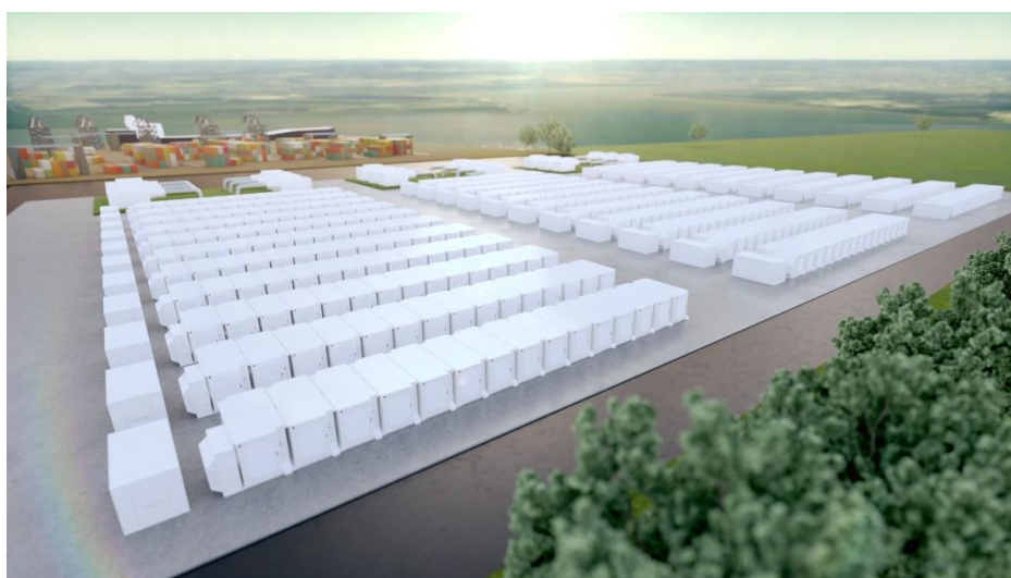
Figure 2: Artist's impression of the proposed 320MW/640MWh Gateway BESS site, one of the world's largest battery projects (source: intergen.com)
